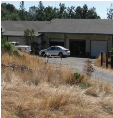
DEFENSIBLE SPACE NONCOMPLIANT
